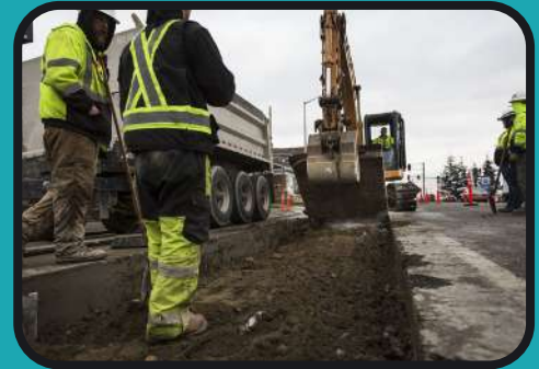
*Common demolition to remove water mains.
